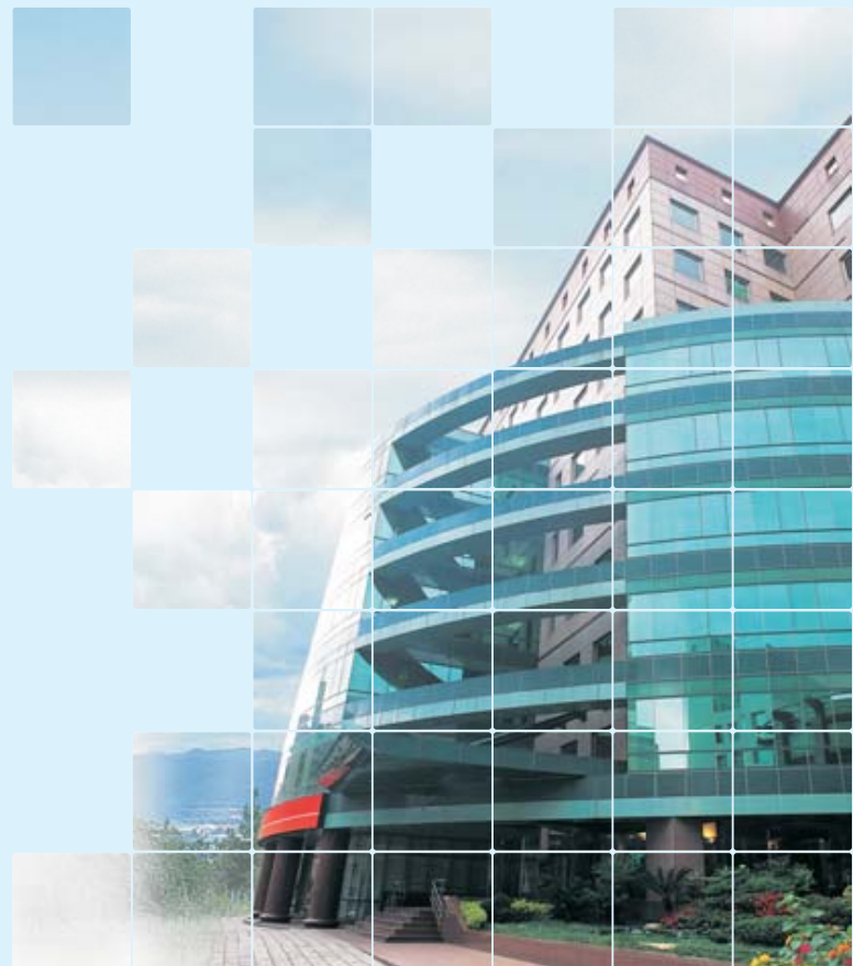
Delta Headquarters Entrance
