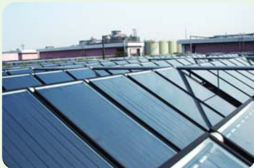
Solar Water Heating Systems
