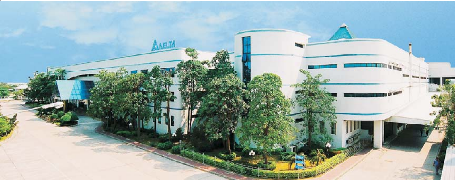
Power Supply Plant, Thailand
