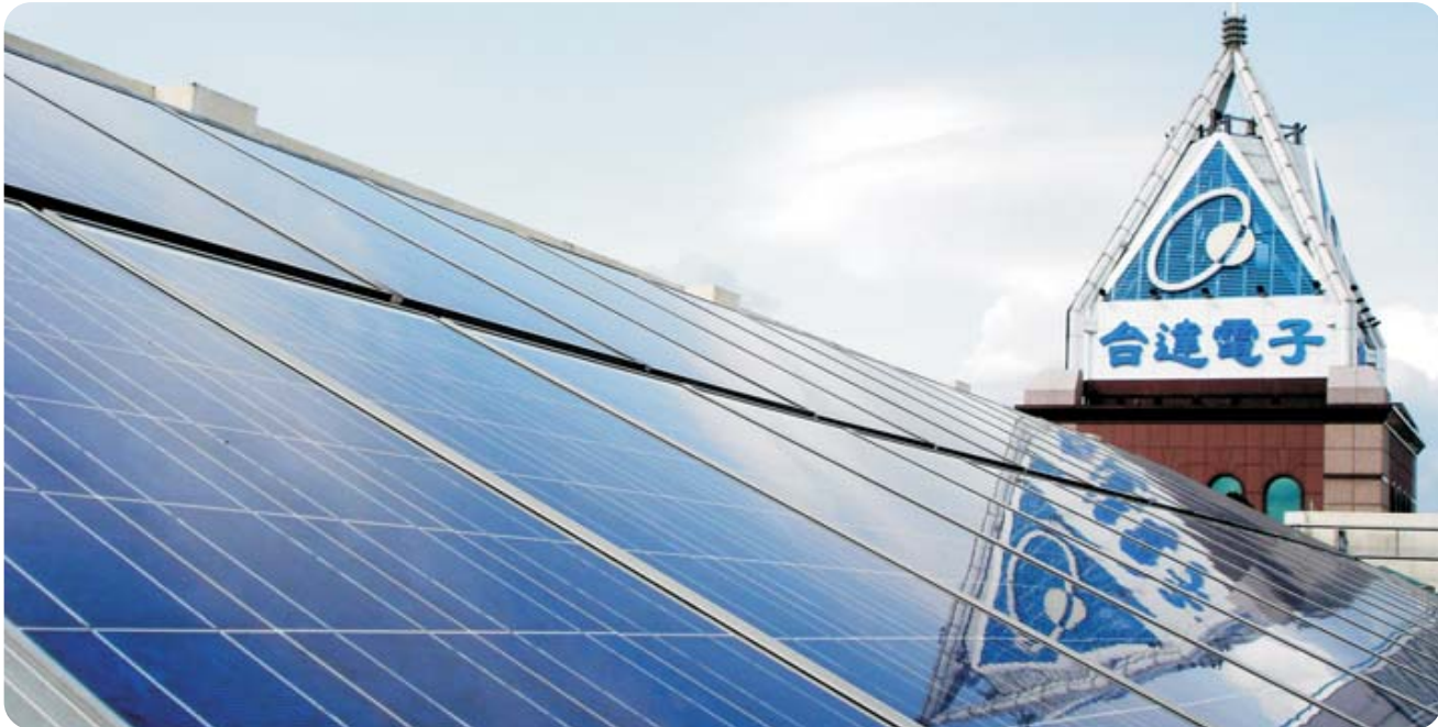
Solar Panels on the Rooftop of Delta Headquarters
