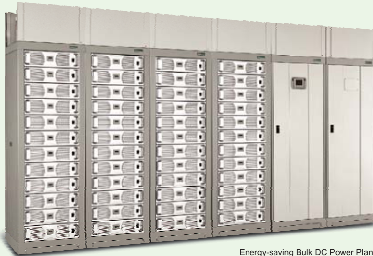
Energy-saving Bulk DC Power Plant
