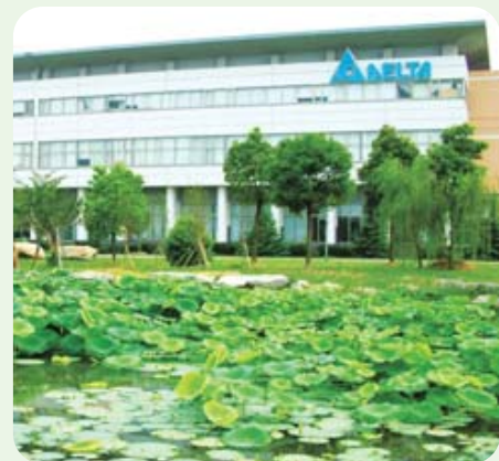
Plant Site Landscaping
