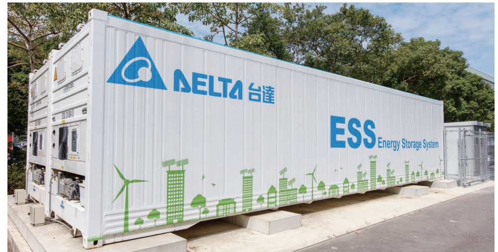
Delta's energy storage system balances renewable energy output and strengthens climate resilience
