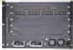
Chassis Switch Systems
