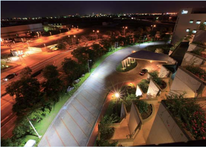
Delta's LED lighting solutions illuminate the Tainan Science Park.
