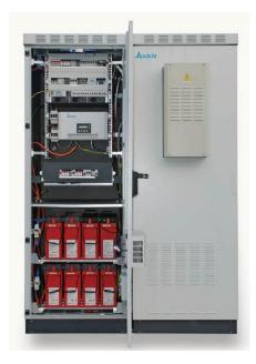
Delta's new RenE-OutD 8700-48 renewable-hybrid solution provides the network site power with any combination of AC grid and diesel generator power with renewable solar or wind energy sources. The RenE-OutD 8700-48 is based on the OutD cabinet with various climate management options for the different environments worldwide.
