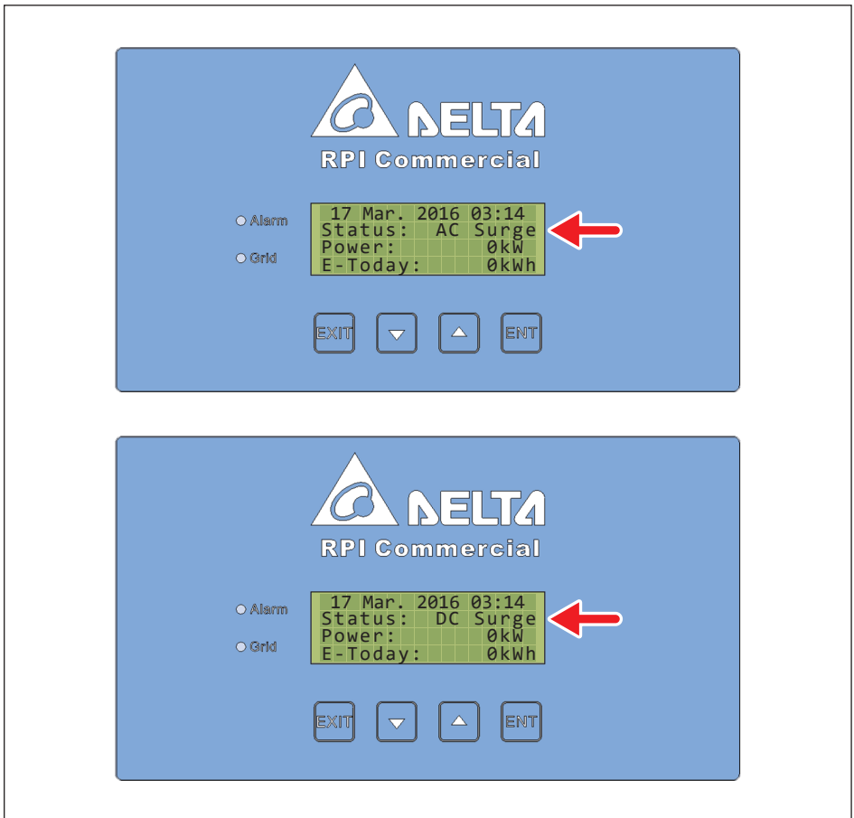
Figure 5-4: Display Indicating AC and DC SPD failure
