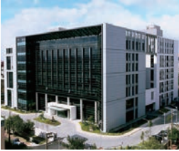
Taoyuan Technology Center (Green Building)
