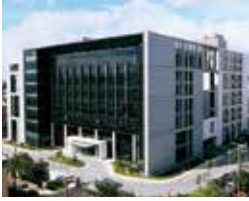
Taoyuan Technology Center (Green Building)
