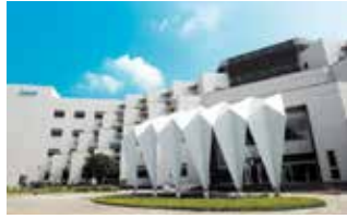
Tainan Plant (Diamond-rated Green Building)
