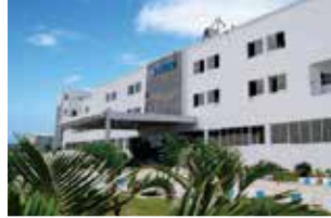
Rudrapur Plant (Green Building)
