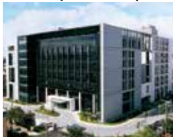
Taoyuan Technology Center (Green Building)
