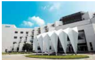
Tainan Plant (Diamond-rated Green Building)
