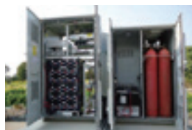
Construction of the first Telecom tower in India which relies on fuel cells for electricity
