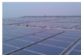
Installation of integrated solar energy system with a capacity of 20MWp in a large paper manufacturing company
