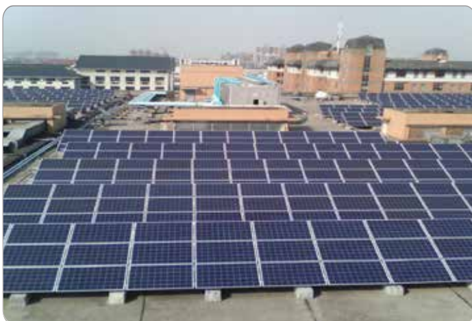
Wujiang Site installed 2.177MWp Solar PV systems.
