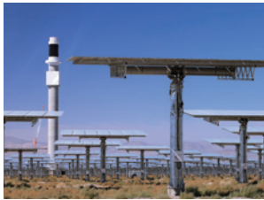
Solar tracking systems for a power plant in the U.S.A.
