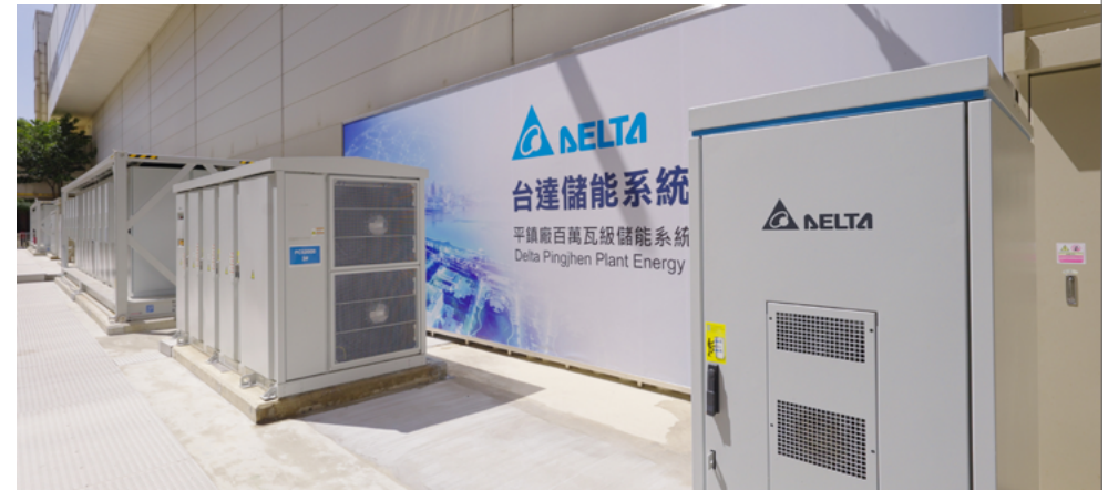
The 5MW energy storage system at Delta's Pingjhen Plant.
