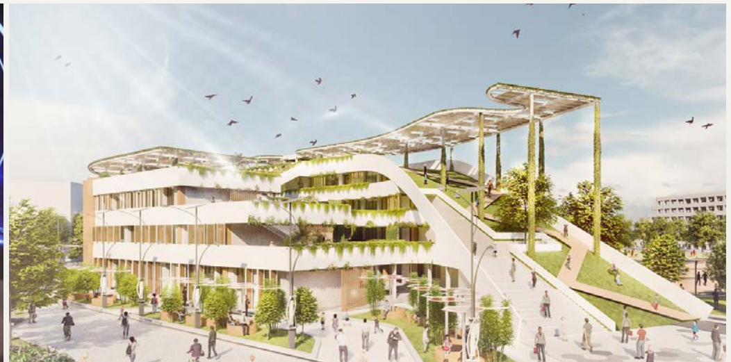
The first-prize entries for the zero-carbon upgrading competition titled "Guangzhou Public Utility Technician College Club Complex" was "Zeroner - Breathing Paradise" by Tianjin University. The work uses vertical greening to achieve passive cooling of the building. The photovoltaic system on the surface of the building creates a continuous and comfortable shady corridor. The movement flow strengthens the connection between the two shapes and makes the space more interesting.
