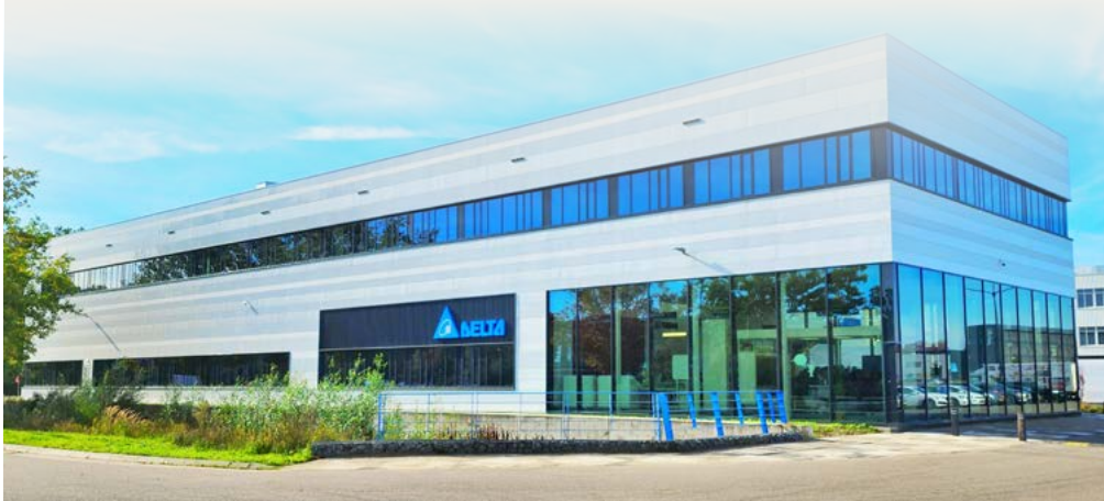
Delta's LEED Gold-certified green building at the Automotive Campus in Helmond, the Netherlands.
