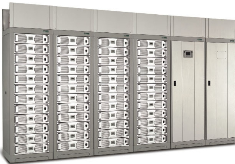
Bulk DC Power Plants
