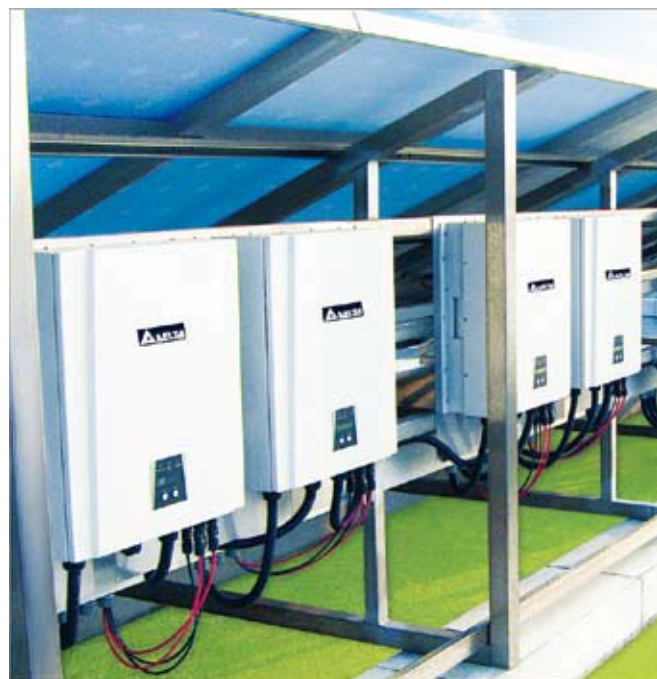
Photovoltaic Inverters Installed under Solar Panels
