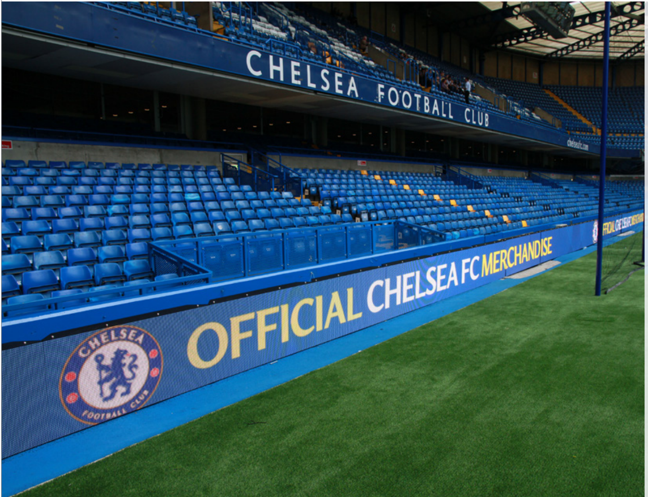
• Delta's LED walls installed at Chelsea Football Club's stadium at Stamford Bridge
