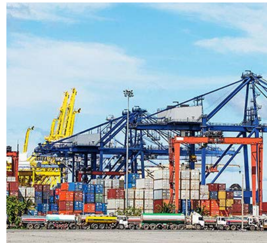
Frontier container terminals in Eastern China implementing Delta's Energy Regenerating Solution to increase the re-use rate of energy.
