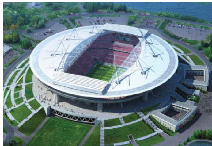
Delta's UPS ensures safe functioning at Zenit Arena facility.
